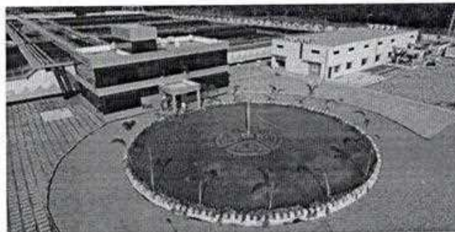
Fig.1.View of STP Kanchanwadi
